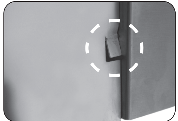
Fig. 27-3 Tab slightly bent in for clearance
